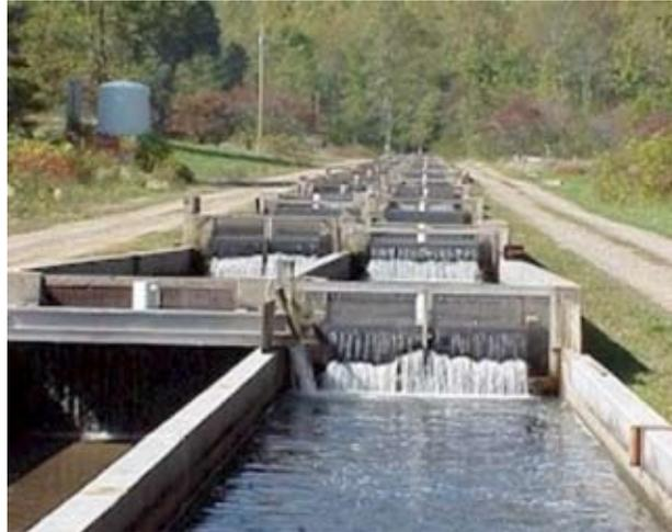
Figure 4. A raceway flow-through system for trout culture.
