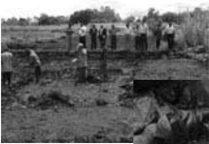
Pond construction at the Sagana Fish Farm.
